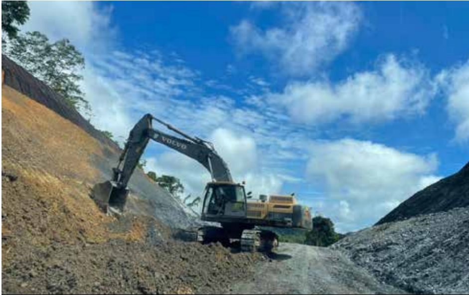
Slope cutting on Baleh Bridge/Pelagus Resort road
