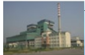
Mukah Coal-Fired Plant (270MW)
