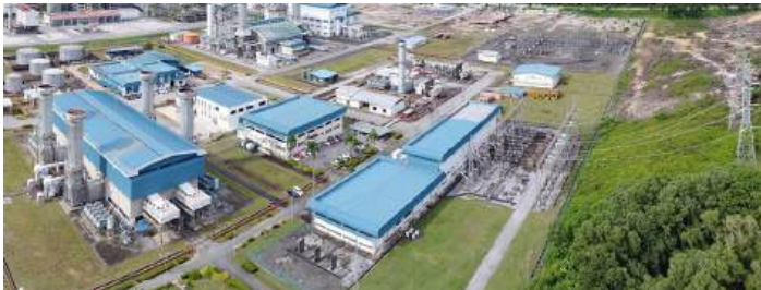
Bintulu Gas-Fired Power Plant
