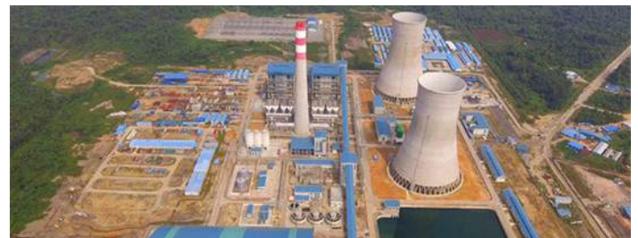
Balingian Coal-Fired Power Plant
