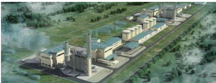
Tanjung Kidurong Combined Cycle Power Plant
