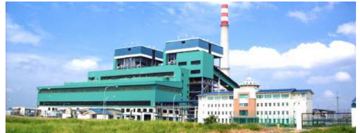
Mukah Power Plant
